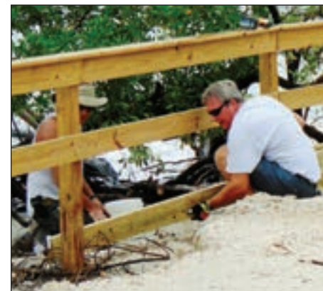
A pair of Department of Public Works employees add a breakwater barrier to the bottom of a fence along the edge of the roadway located on the east end of Sanibel
